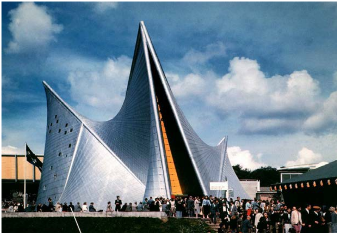
Image No.4 – The final structure of the Philips Pavilion for International Expo 58, also demonstrating the hyperbolic paraboloids originally used in Metastaseis .
